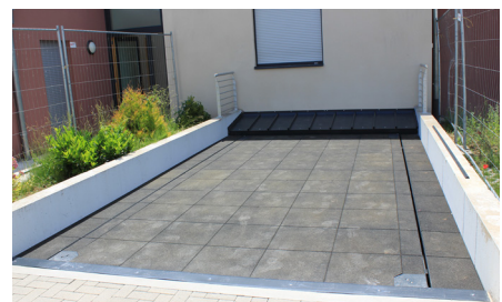
Rubber covering in stone structure (3 cm thick)
